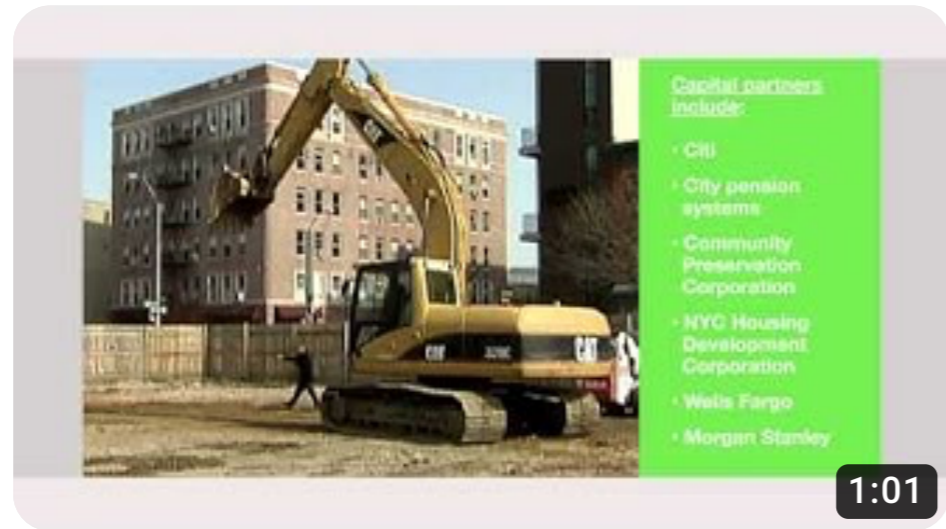
City Scoop: Developers Build Affordable Housing, Small Business First Initiative, Ful...
