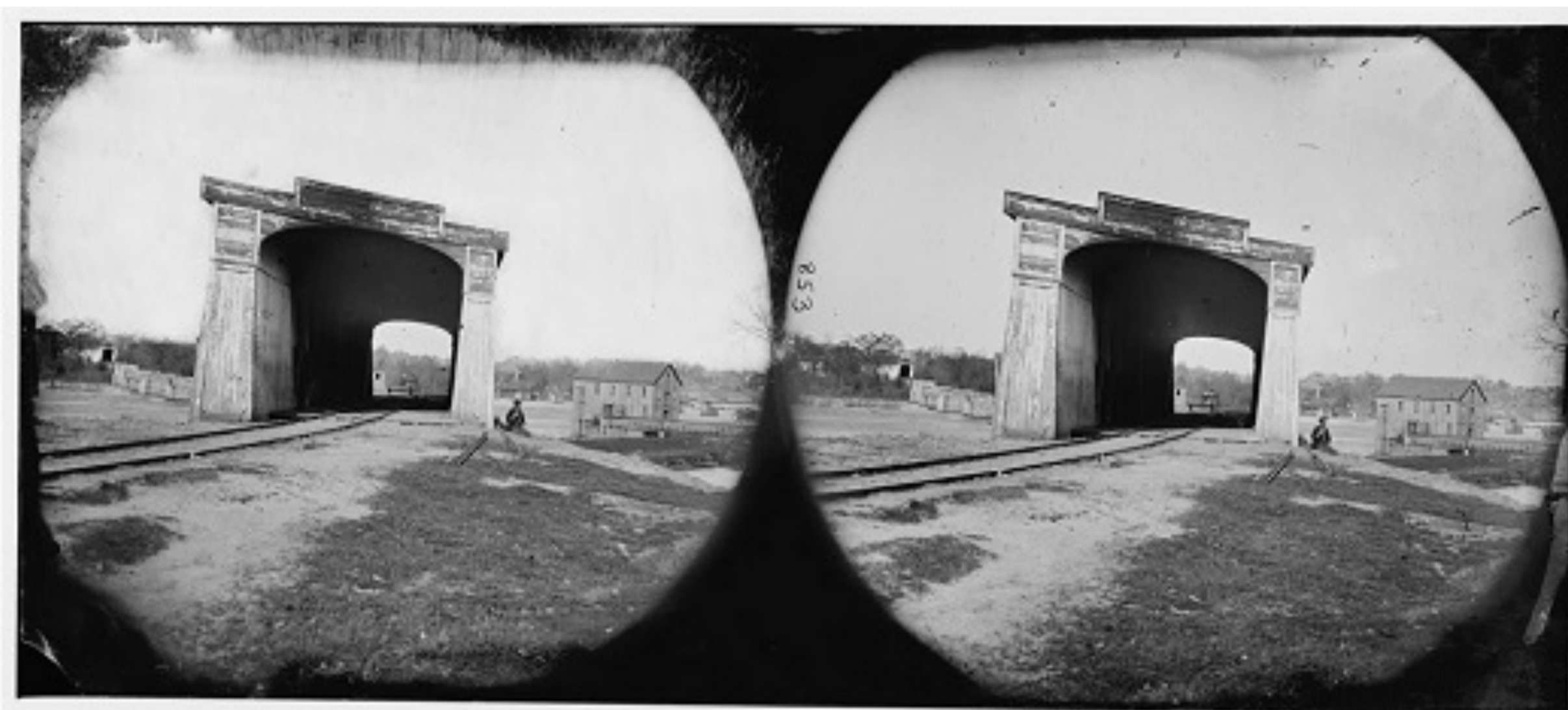
Richmond, Va. Ruins of Richmond & Danville Railroad Bridge . Alexander Gardner, photographer, [1865]. Civil War Glass Negatives and Related Prints . Prints & Photographs Division
