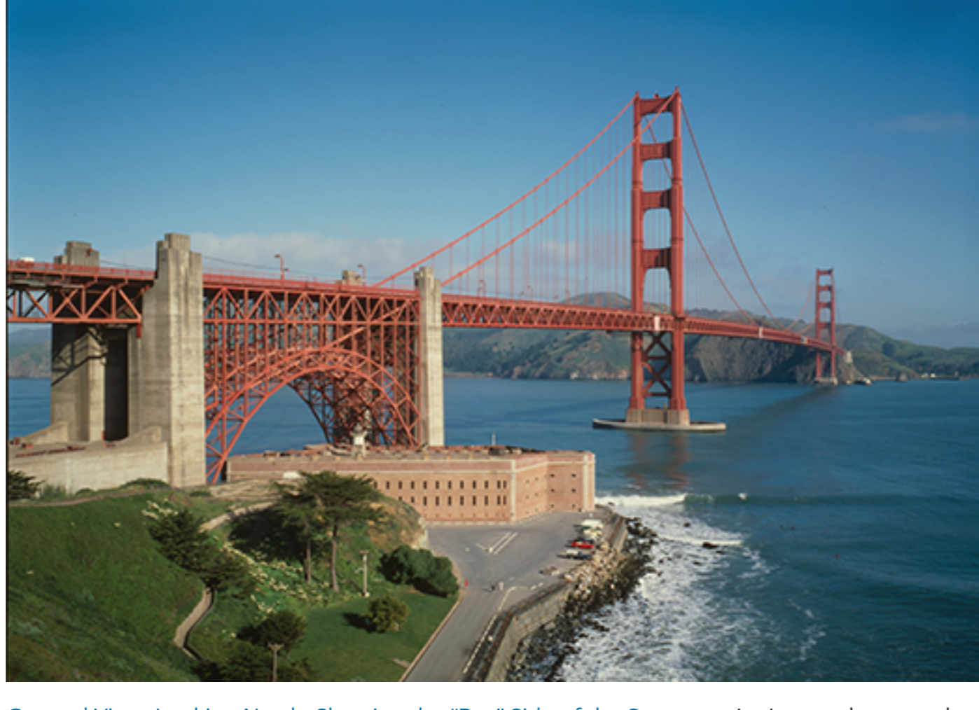
General View, Looking North, Showing the "Bay" Side of the Structure. Jet Lowe, photographer, 1984. Golden Gate Bridge, San Francisco, California. Historic American Buildings Survey/Historic American Engineering Record/Historic American Landscapes Survey. Prints & Photographs Division
